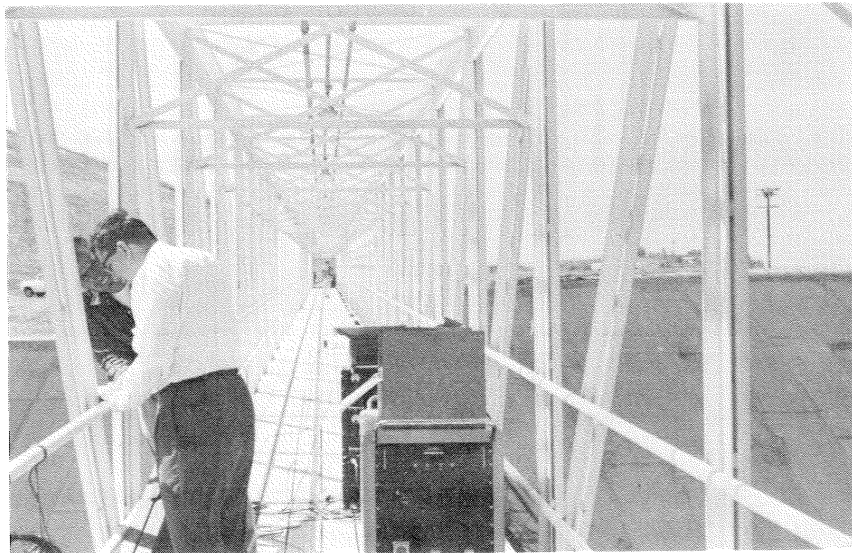
VIEW OF BRIDGE, LOOKING TOWARDS DAM
