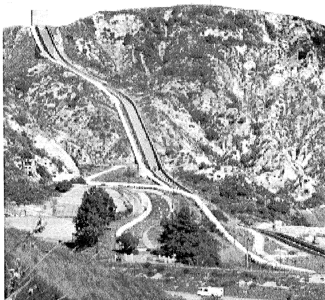
Figure 5. Photograph in northern Granada Hills showing the two sets of channels and penstocks representing the terminations of Los Angeles Aqueducts 1 (left) and 2 (right).
